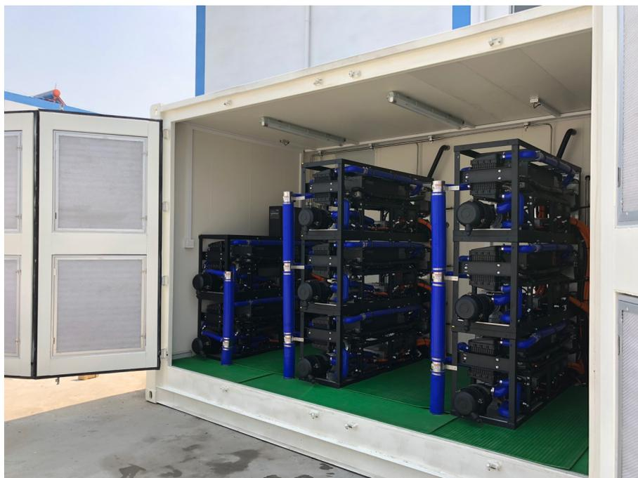
Horizon 30kW FC stacks installed in the 200kW system
